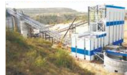
YIDONG COAL GROUP COAL PREPARATION PLANT
