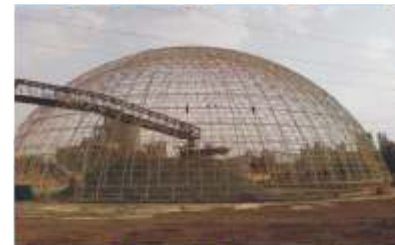
STORAGE SILO OF BIRLAR CEMENT PLANT, INDIA
