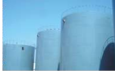
SINOPEC STORAGE TANK
