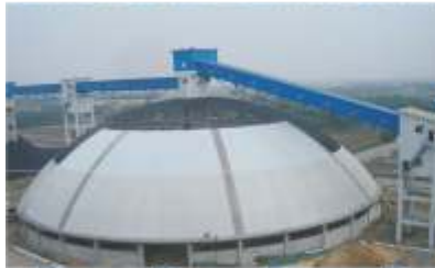
HUAINAN MINING BUREAU CAPTIVE POWER PLANT
