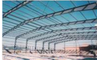
DONGGUAN DONGYI STEEL STRUCTURE
