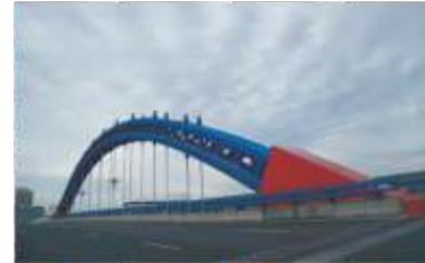
HENG SHUI YUHUA STREET CROSSES BEIJING-KOWLOON RAILWAY BRIDGE
