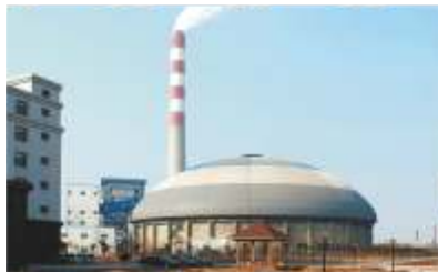
JINING POWER PLANT COAL STORAGE DOME
