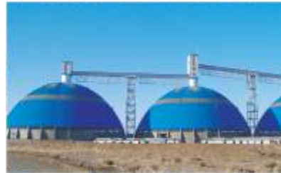
OPEN-PIT COAL STORAGE DOME
