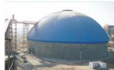
INDIA CEMENT PLANT COAL STORAGE BUNKER
